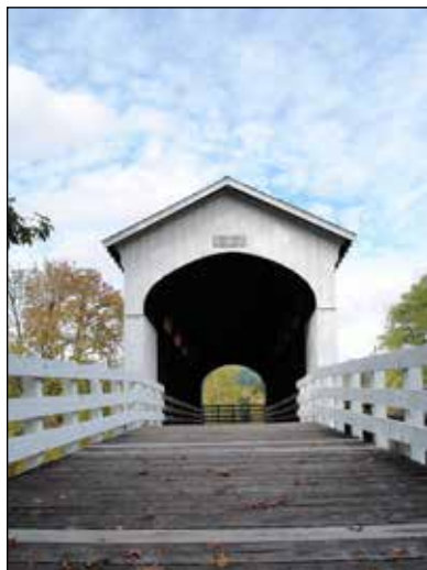
Currin Covered Bridge
