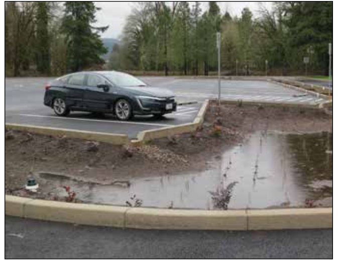
Storm Water Drainage After a Heavy Rain, Hendricks Bridge
