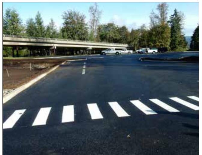
Newly Constructed Walkway to Hendricks Bridge Boat Ramp (West Viewpoint)
