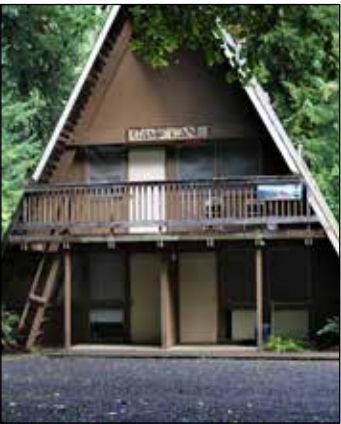
Camp Lane A-Frame Cabin
