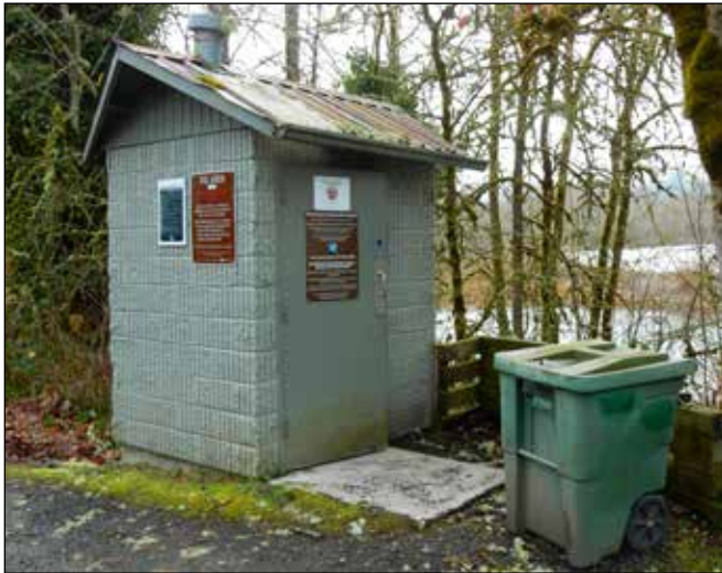
Public Restroom at Bellinger Landing County Park
